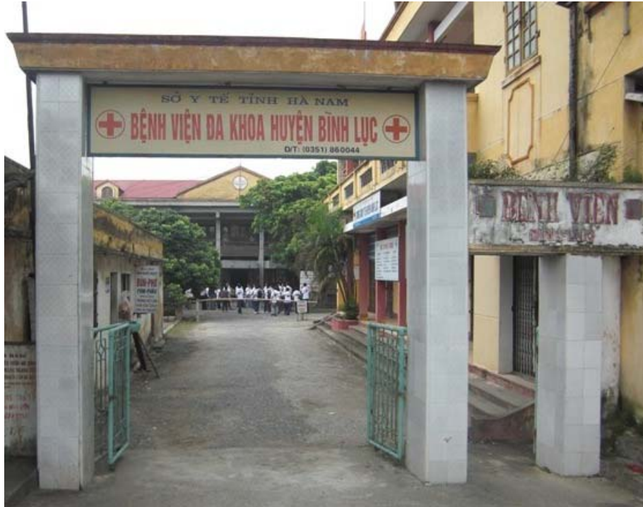
(Above) Bin Luc Hospital is a case study for the SMP Global Leaders to build the Public-Private Partnership framework. Photo: Panos Vrahiotis
